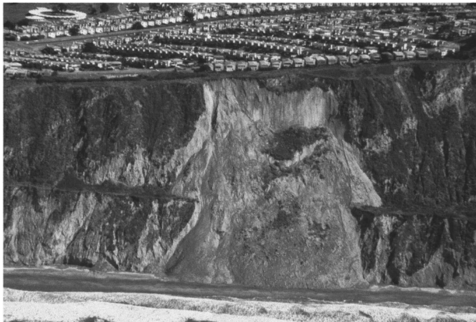
Fig. 2. Failure of bluffs in Daly City caused by 1989 Loma Prieta earthquake
