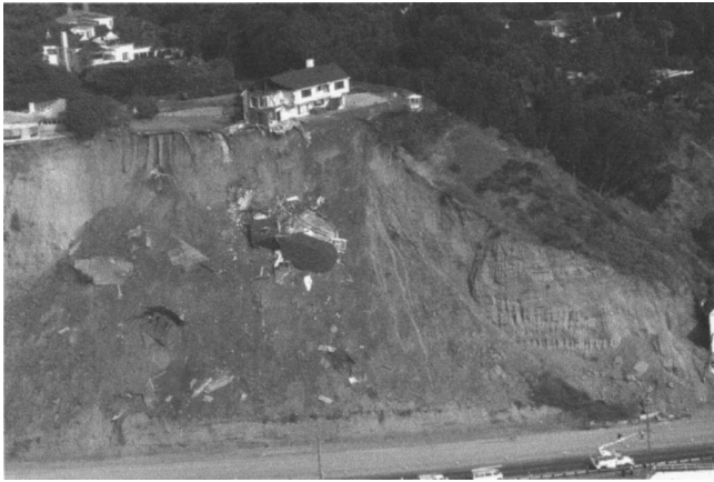
Fig. 3. House destroyed in bluff failure at Pacific Palisades during the 1994 Northridge earthquake
